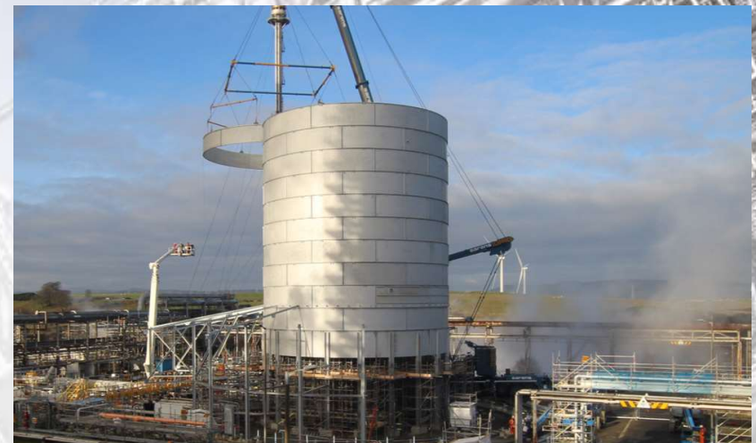
Final ring being lifted into place
