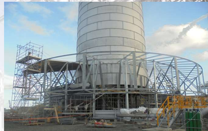
Noise-reducing-shroud installation underway
