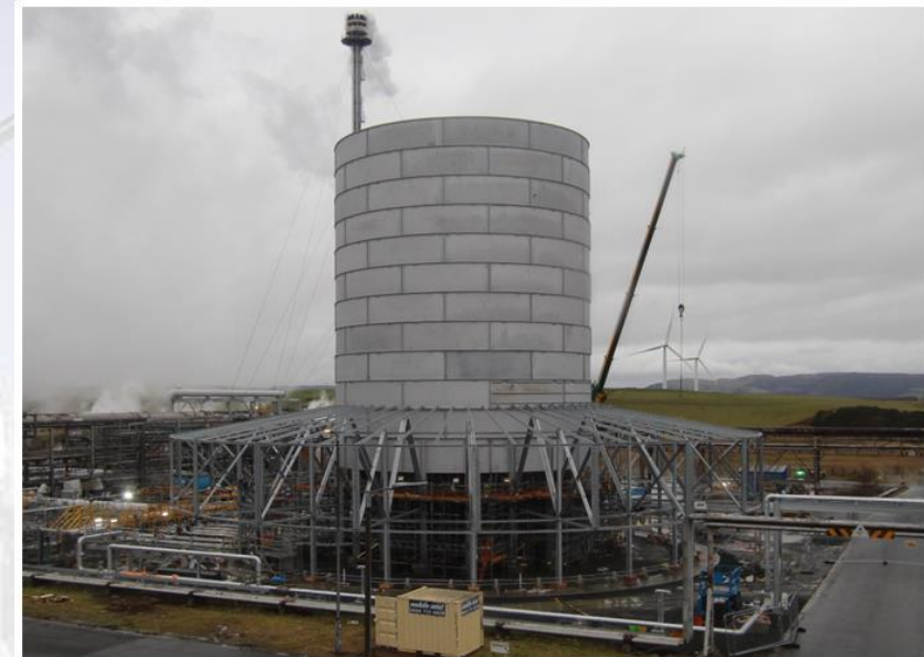
Shroud structural steel work progressing
